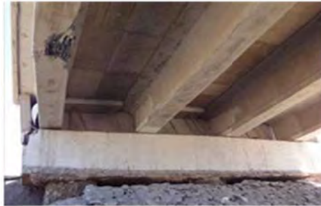
Fig. 4.7 Damage in Chada Bridge with no diaphragm.
